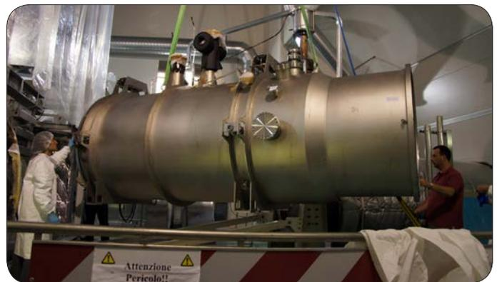
Figure 3. Installation of the first cryolink at Virgo's North End building, summer 2014.
